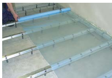
Installation, floating 22 mm chipboard
